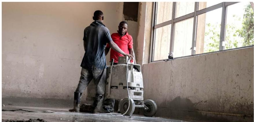
Two machine operators work on a construction site, handling terrazzo flooring. Using wet methods significantly reduces airborne silica dust generated during milling or grinding of silica-containing materials.
