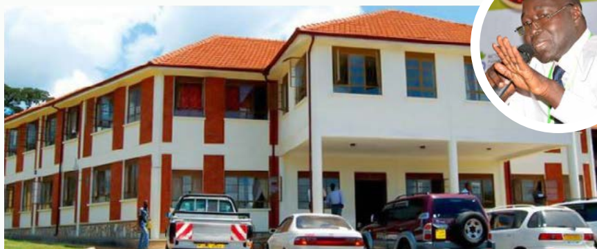
Wakiso district administration block. In set, Dr. Richard Kajura, the pioneer community Lab Director.
